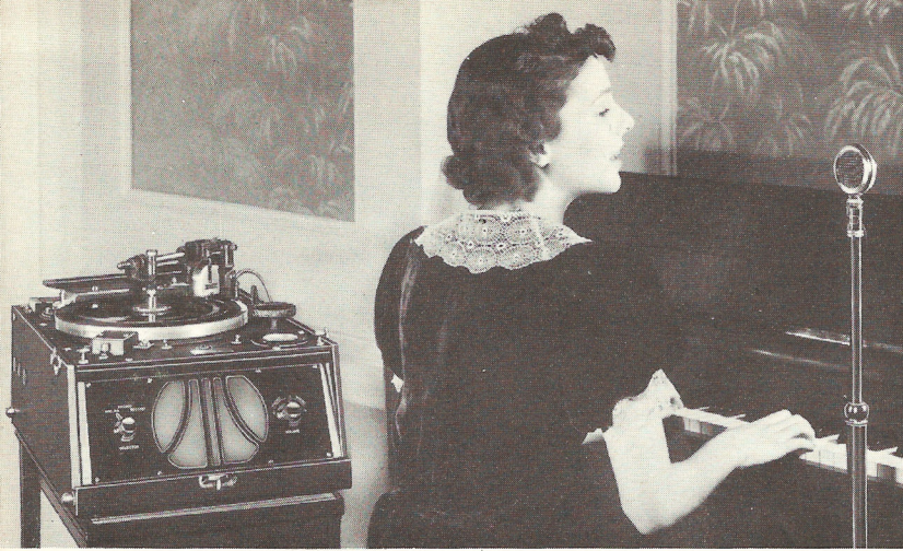
With a view to making the Chicago Conservatory as complete as possible in every detail, a Presto Model Recorder, of the type used in ninety-one Broadcasting Stations, has been installed. This instrument is especially designed for making records which may be played with a steel needle on any phonograph.
