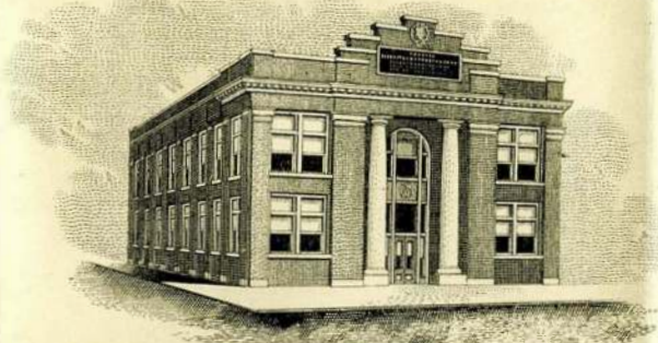
EL PASO CHAMBER OF COMMERCE BUILDING
