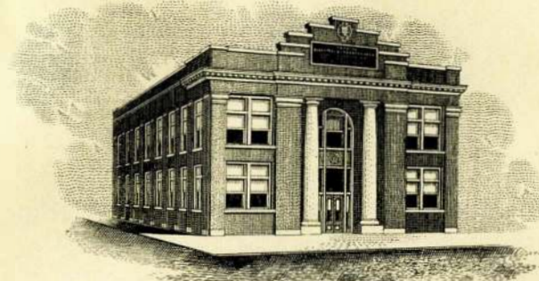
EL PASO CHAMBER OF COMMERCE BUILDING
