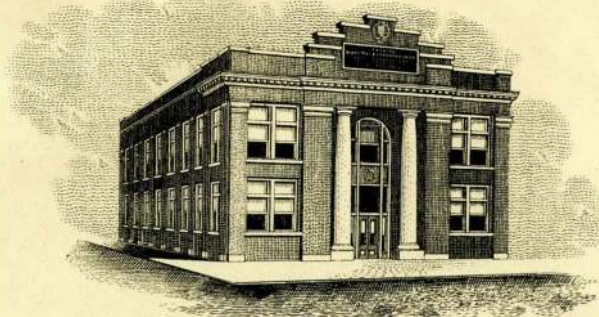
EL PASO CHAMBER OF COMMERCE BUILDING
