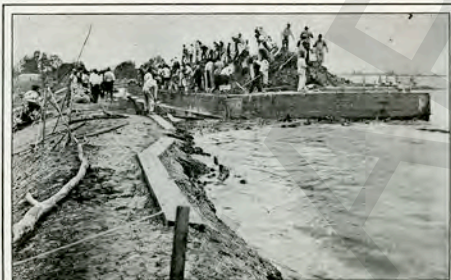
THE BARGE THAT SAVED THE DAY Loaded with dry earth from a distance, it arrived "just in time to save St. Delphine Levee, May, 1922." More than half of all the Mississippi levees are in Louisiana.
