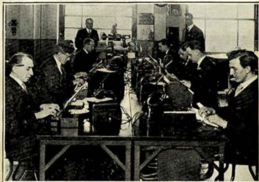
OPERATING THE EUROPEAN END OF THE WORLD'S FAST- EST CABLE, DESIGNED TO TRANSMIT AS MANY AS EIGHT CABLEGRAMS AT THE SAME TIME.
