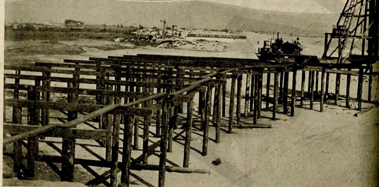
Glimpse of rapid progress in pier building at Ensenada, taken July 15th. Insert, commencement of pier snapped July 4th
