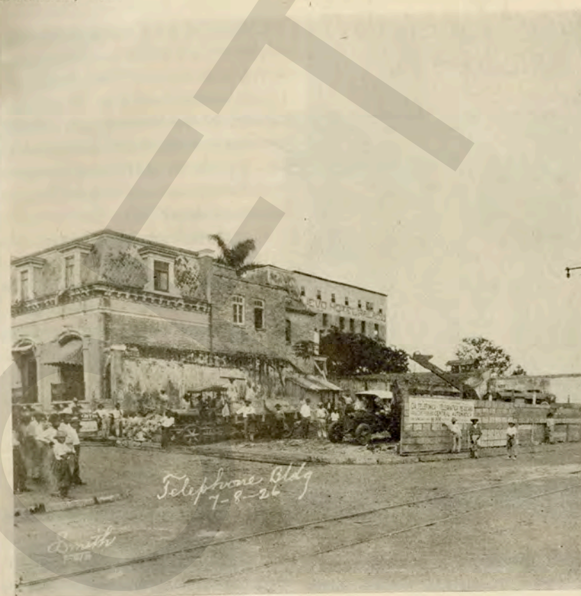
Excavation for Central Office Building at Tampico, July, 1926.
