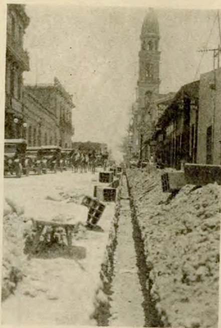
Installation of subway of 18-way ducts in Calle de Estado between Muelle and Empresa. Tampico, June, 1926.
