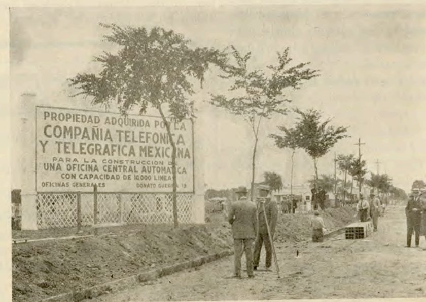
Big Sign on Property of the Company. Also First Clay Ducts Unloaded.
