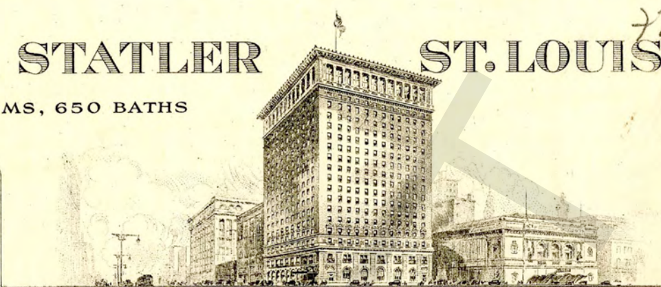
Washington Avenue at Ninth and Saint Charles
