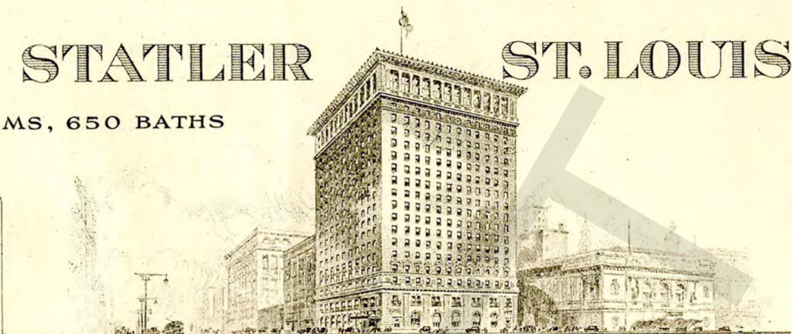
Washington Avenue at Ninth and Saint Charles
