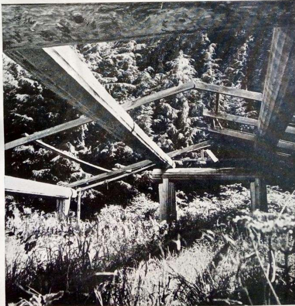
Above, detail showing the fluting caused by the stripping off bark by means of an adze. Below, framework of a Community-house.
