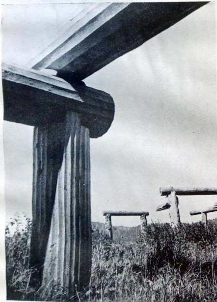
Posts and beams of Community-houses Mamallilacoola, British Columbia.
