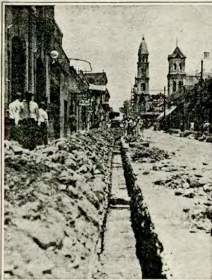
TAMPICO OPTICAL CO. Excavating for Underground Telephone-Conduit System at Tampico
